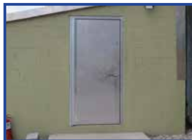
Mechanical Room Flood Door (PD-525)
