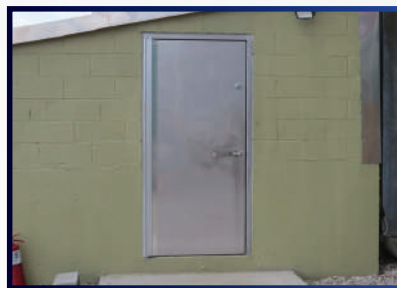
Mechanical Room Flood Door (PD-525)
