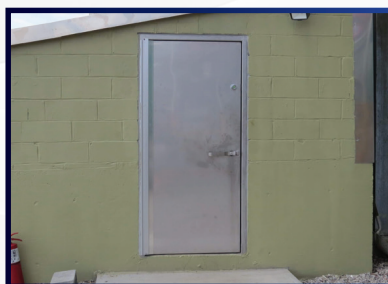
Mechanical Room Flood Door (PD-525)
