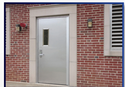
Fired Rated Flood Door (PD-522)
